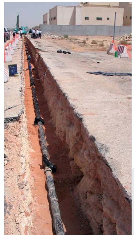
Pipeline construction in Riyadh, Saudi Arabia
