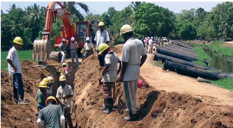
Pipeline construction in Sri Lanka
