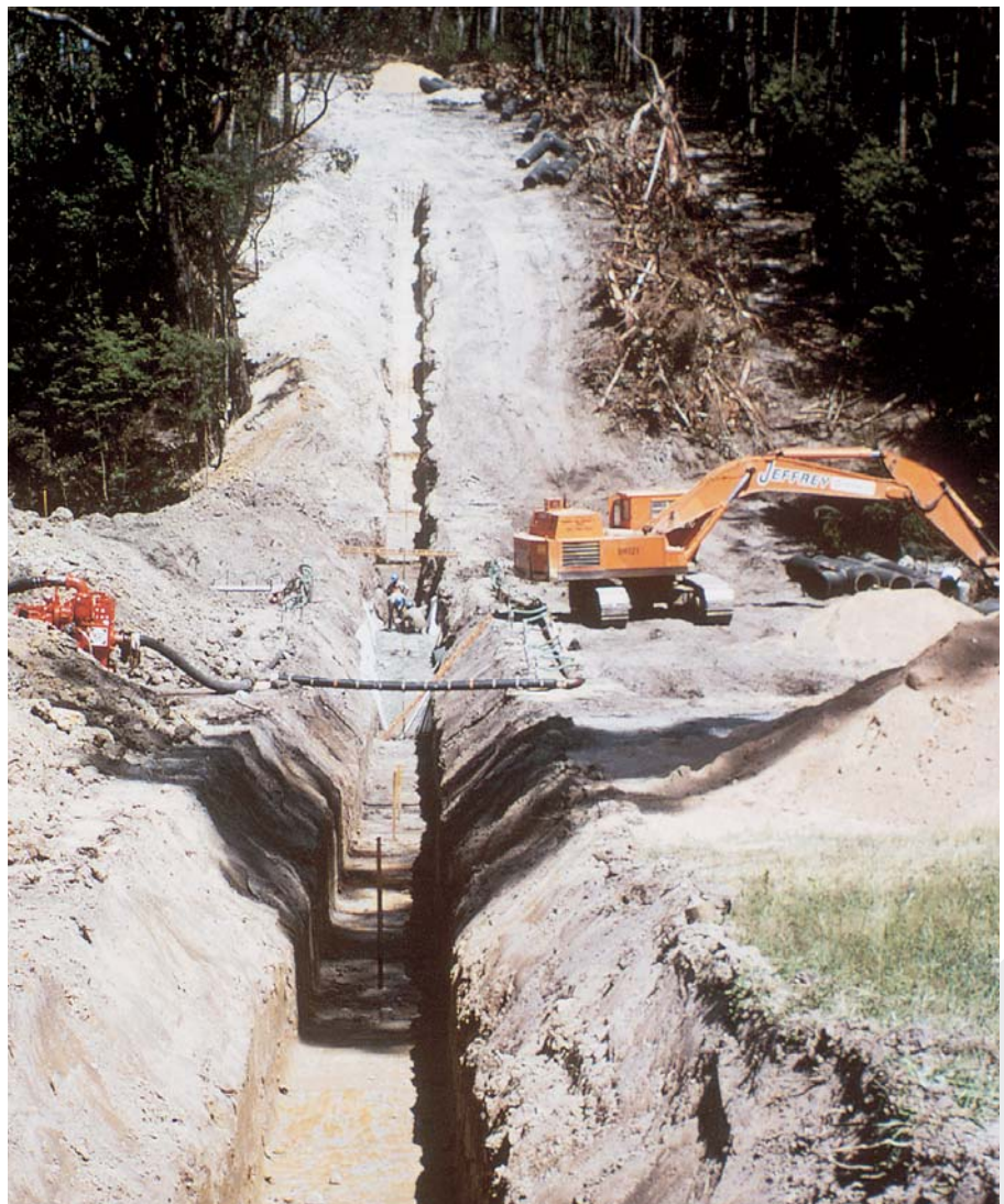
Trench incorporating gradient anchors
