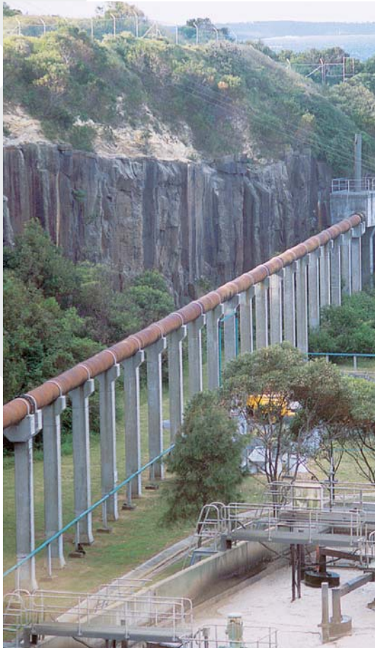
800mm pipeline on columns, supported at 6 metre centres
